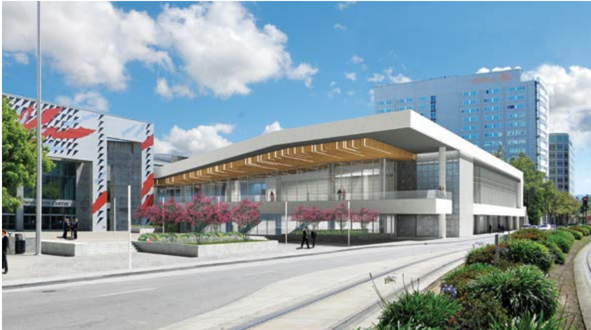
San Jose McEnergy Convention Center, California
